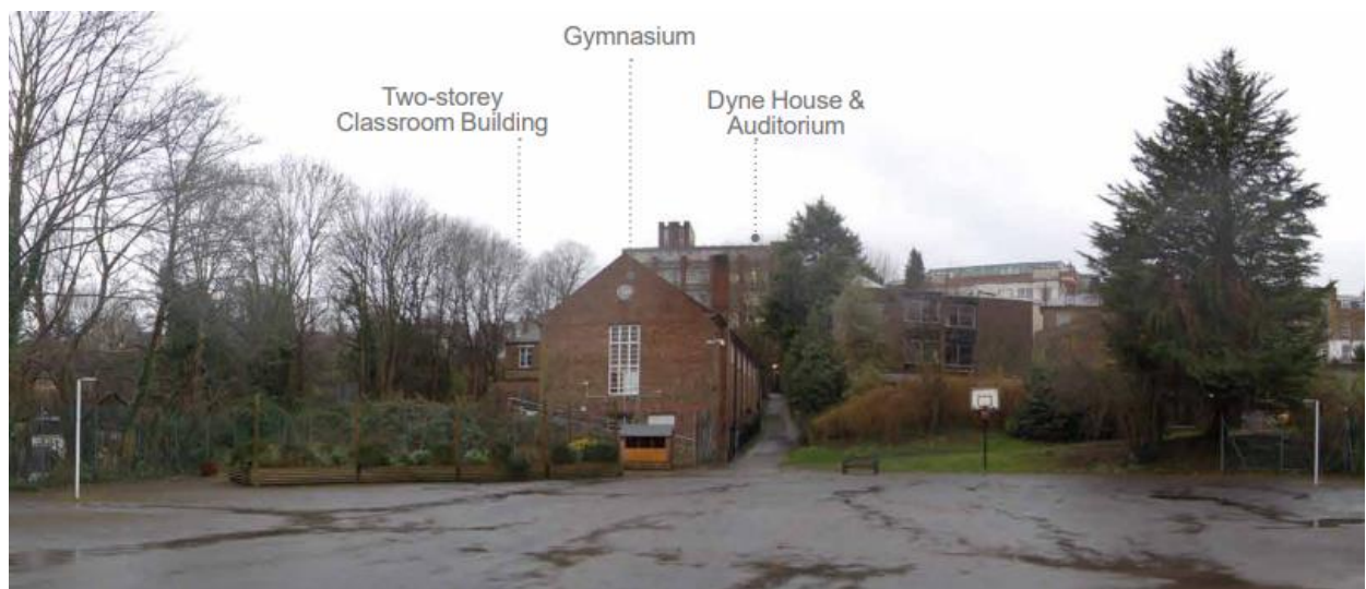
Photo of Rear Elevation
